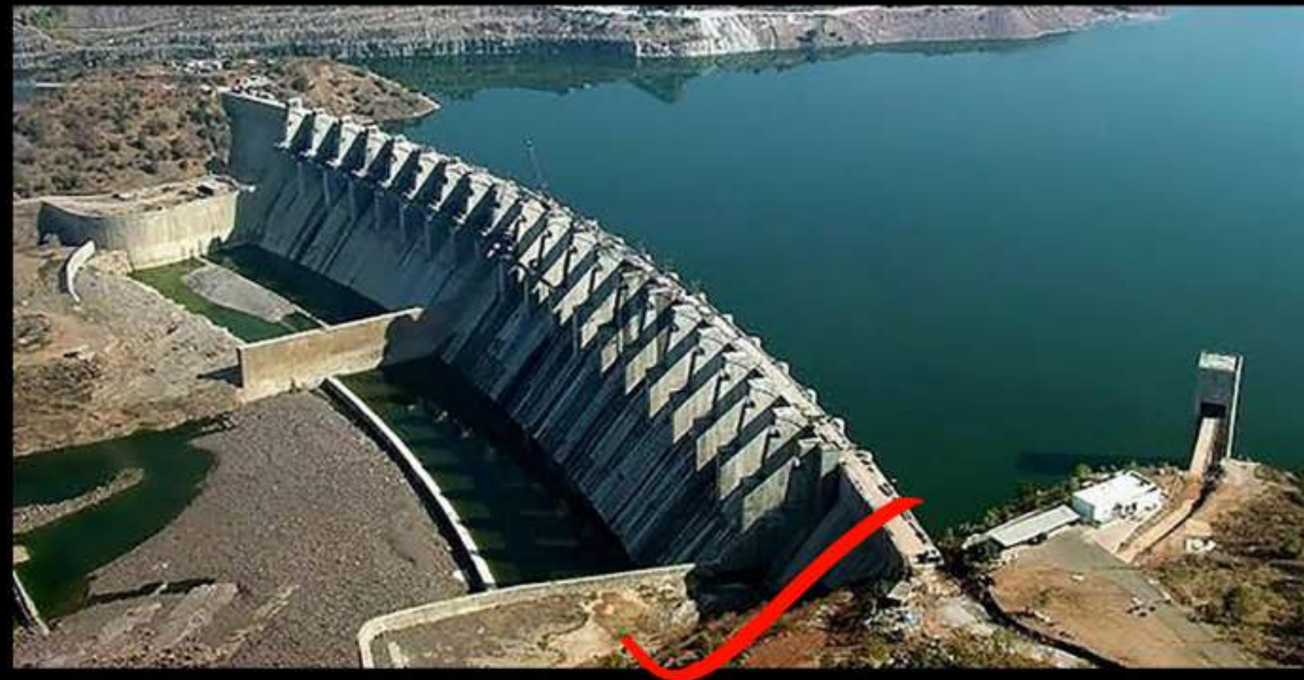
Indira Sagar Dam
